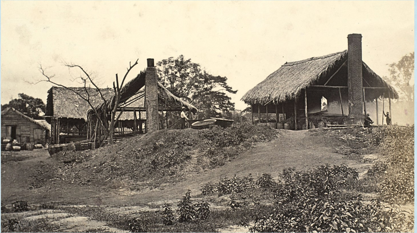
A pair of boiling Houses where raw pitch is melted. Close to the Pitch Lake, La Brea, Trinidad, 20 Jan 1880 RCIN 2580463 - By Todd-White Art Photography & The Royal Collection Trust, UK
